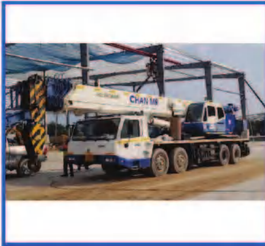
Truck Crane 1 unit
